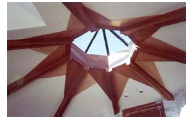
A unique octagon ceiling with skylight Maple and Cherry Trim
